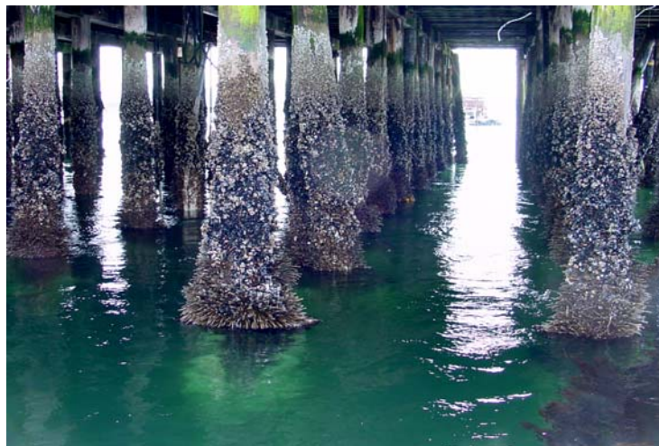
Figure 5. Piling supporting the Fort Ward wharf in Rich Passage, Washington. The wharf's deck is constructed of ACZA treated 3" x 8" lumber.
